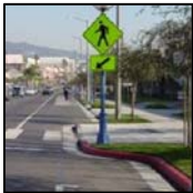
Install mid-block curb bulb
