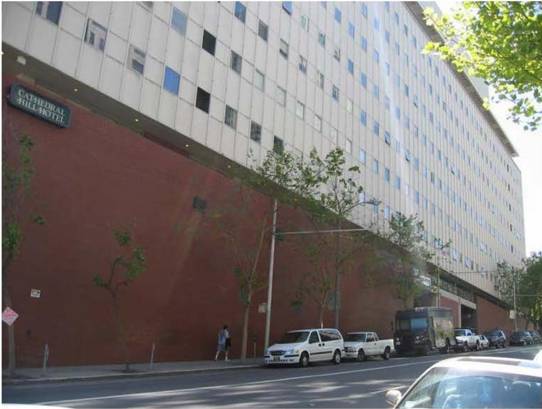
View looking southwest from Post Street
