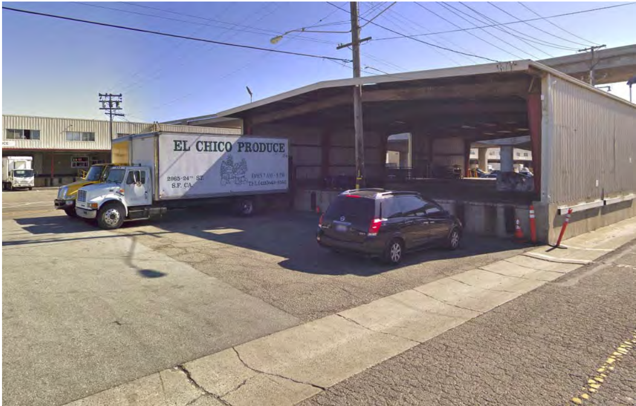
Figure 50: A typical (off-street) freight loading instance. Source: Google Street View, 2018.
