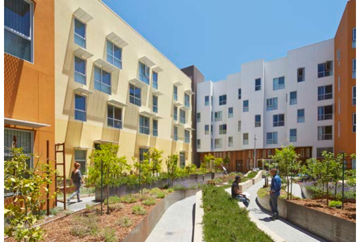
Bayview Gardens. Photo: Bruce Damonte
