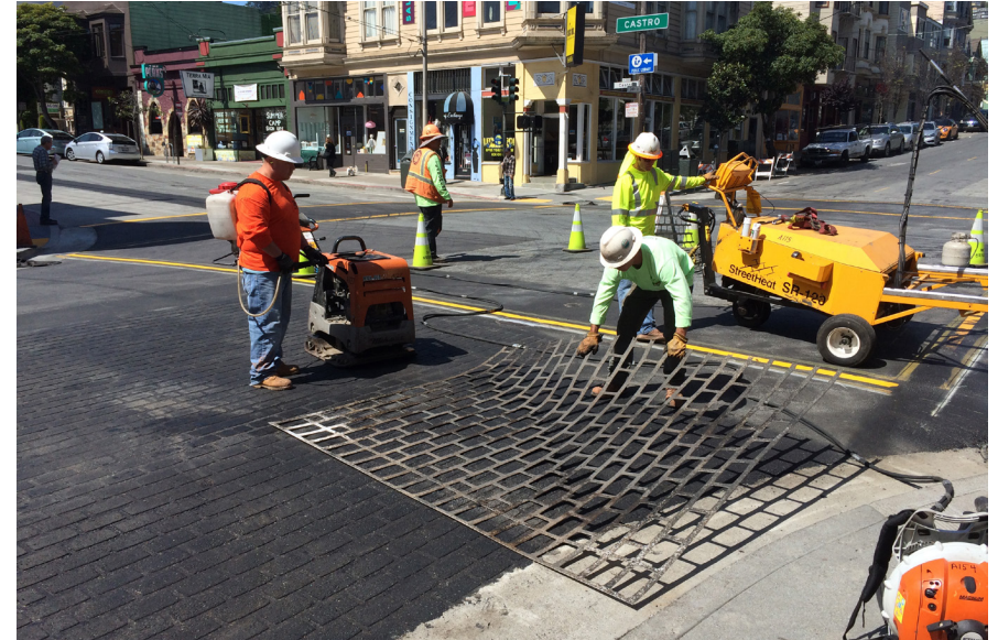
Example of City-installed projects: stamped asphalt crossings.
