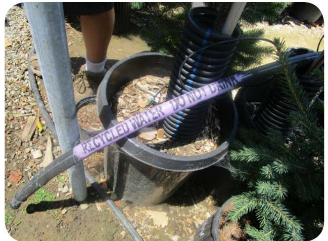
Irrigation frame using recycled water for watering of trees and plants at Our City Forest Street Tree Nursery
