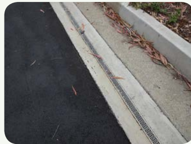
New drainage system for collection of irrigation water for reuse
