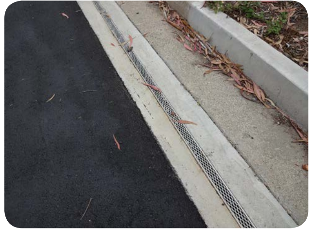
Drains in Presidio Nursery capturing irrigation runoff for reuse
