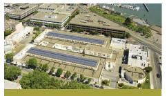
Built in 1951 Only active during wet weather Treats up to 150 MGD during rain storms Located at Bay Street and The Embarcadero
