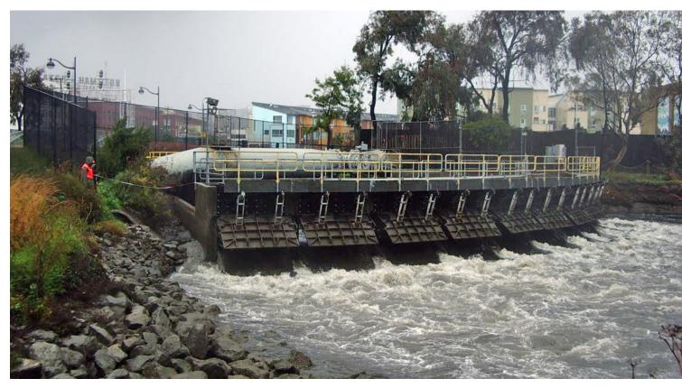
Photo 7.5 Division Combined Sewer Discharge. SFPUC
