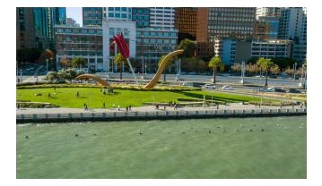
The Embarcadero Seawall is over 100 years old and was designed and constructed before engineers understood how to build infrastructure to survive earthquakes. Most of the seawall is built over "young bay mud," a weak, saturated, and highly compressible marine clay that tends to amplify earthquake shaking. The seawall has aged and settled, and no longer offers sufficient flood protection.
