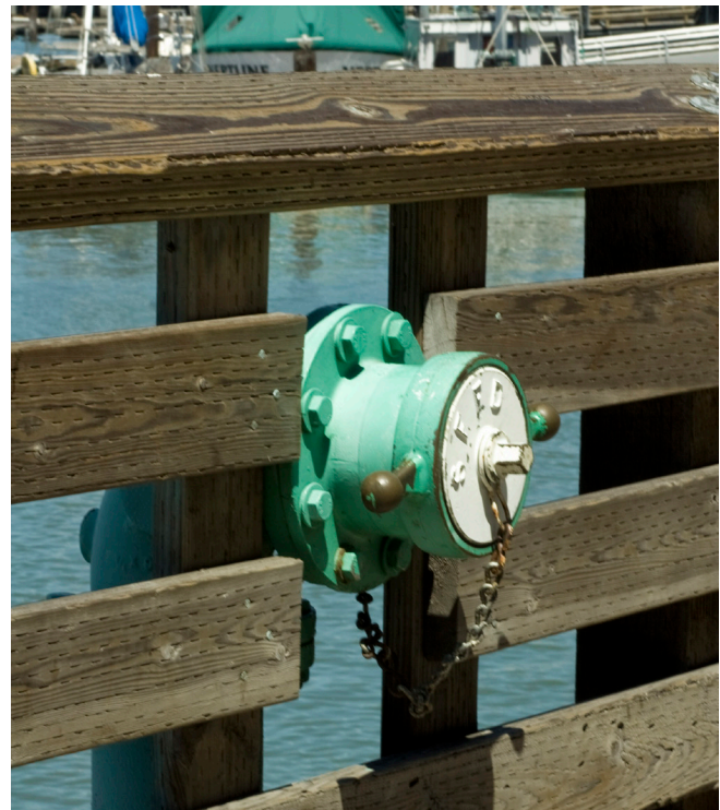
Photo 9.10 Suction connection (Baywater 'fire hydrants'). Jason Randall
