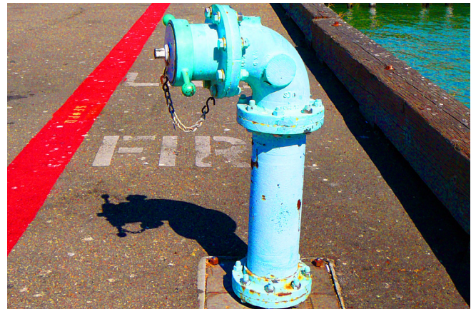
Photo 9.6 High-pressure fire hydrant. Kitty DuKane (CC BY-NC 2.0)
