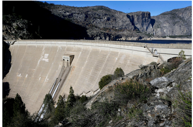
Photo 8.1 Dam at Hetch Hetchy Reservoir. Michael Macor, The Chronicle
