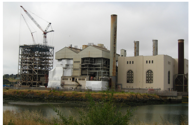
Photo 8.4 PG&E Hunters Point substation. Salim Virji (CC BY-SA 2.0)
