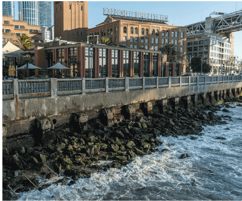
Existing seawall along the Embarcadero. Port of San Francisco
