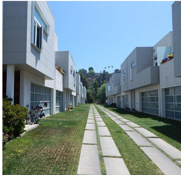
Figure 5.17-2: Permeable and vehicular rated paving is used to maximize pervious surface for stormwater management
