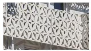
Perforated Metal Guardrail
