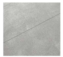
Cast-in-place concrete with silicon carbide and saw-cut joints at pathway
