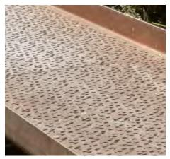
Slip-resistant weathered steel decking at rain garden elevated walkway
