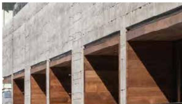
*Board Formed Concrete and Acetylated Wood*
