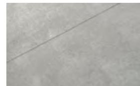
CIP Concrete: Natural Gray w/ Silica Carbide and Water Jet Finish
