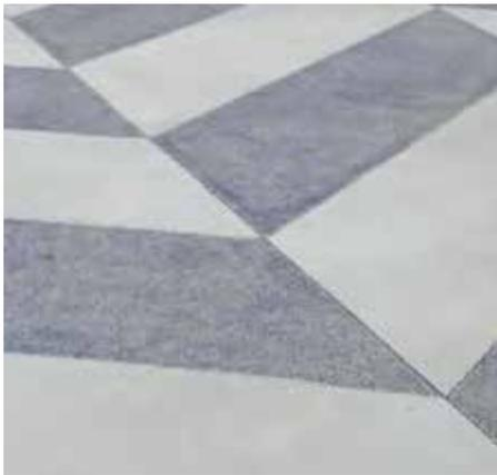
*Contrasting patterns of cast-in-place concrete with seeded aggregate and colored surface pattern at SFPUC Retained Fee Open Space*
