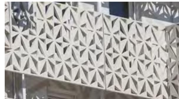
*Perforated Metal Guardrail*
