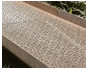
P8: slip-resistant weathered steel decking at rain garden elevated walkway
