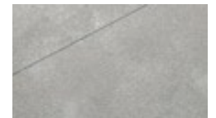
Cast-in-place concrete; medium gray w/ silica carbide and water jet finish
