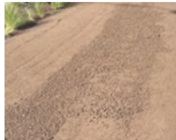
P11: compacted decomposed granite, red-brown pathway mix
