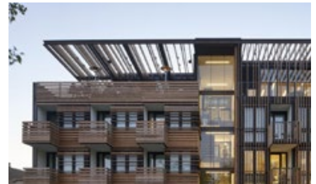
Roof terrace expressed on facade
