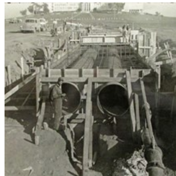
Balboa Reservoir Inlet/Outlet Pipes, 1957
