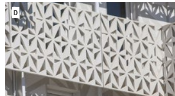
Perforated metal guardrail
