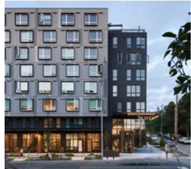
Building entry related to scale of modulation of the facade
