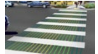
Thermoplastic crossing with custom pattern inlay
