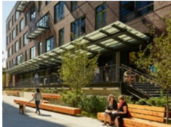
Reservoir Park frontage, shared entry porches
