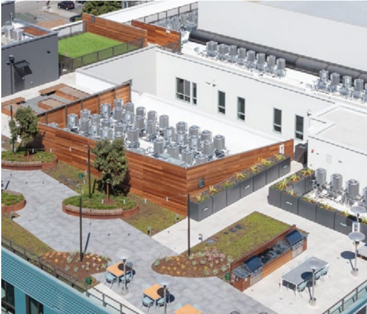
Screening of rooftop mechanical equipment
