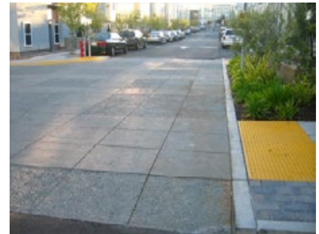
Raised street crosswalk
