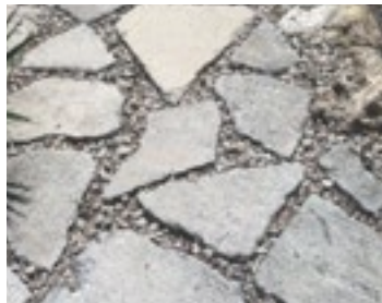
P5: permeable recycled concrete paving salvaged from the existing reservoir concrete slope with gravel joint
