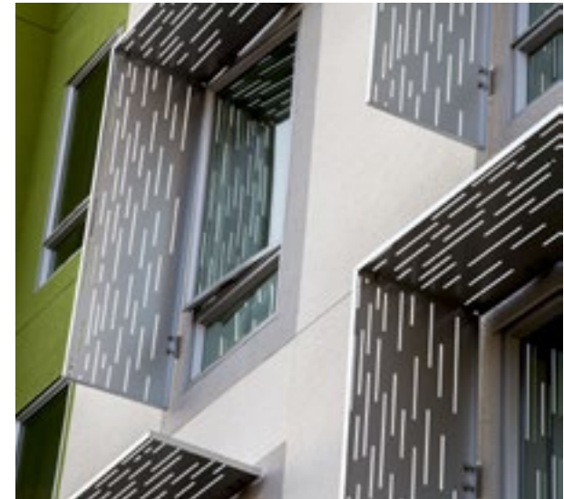
Sunscreens to reduce solar gain
