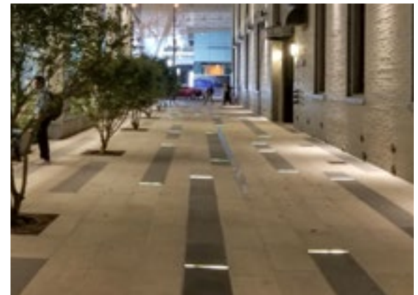
Small, distributed, low-voltage lighting
