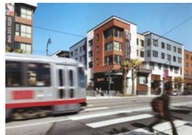
Ocean Avenue mixed-use buildings
