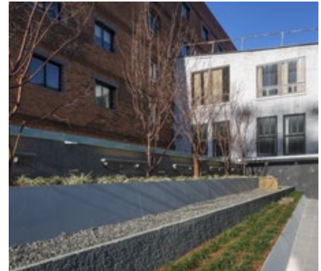
Seasonal stormwater feature in private courtyard
