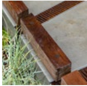
Heavy timber wheel guide and accessible stormwater channel
