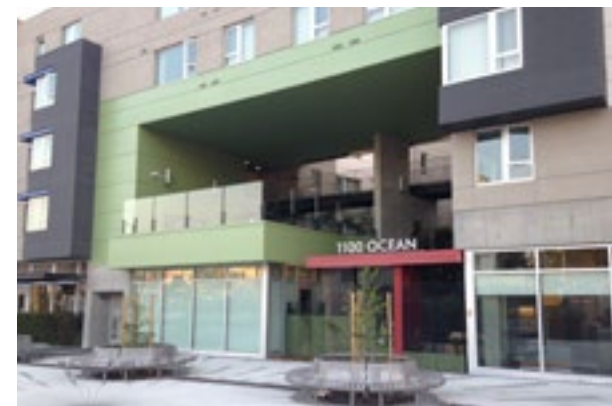
Building allowed to bridge over opening to courtyard
