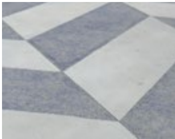
P2: cast-in-place concrete with seeded aggregate
