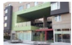
Building allowed to bridge over opening to courtyard
