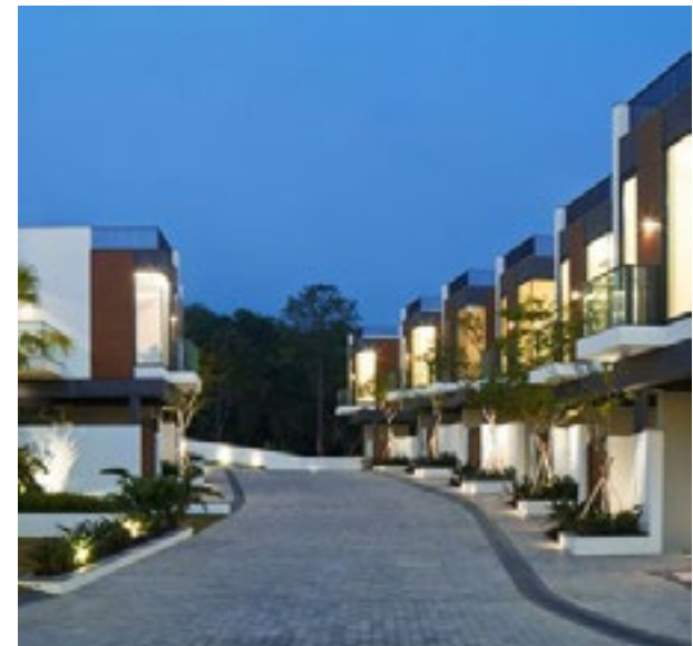
Figure 5.17-4: High quality paving material, planting and accent lighting create a pedestrian environment.
