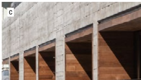
Board formed concrete and acetylated wood
