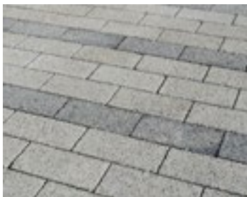
P3: Pervious concrete paving with grind finish
