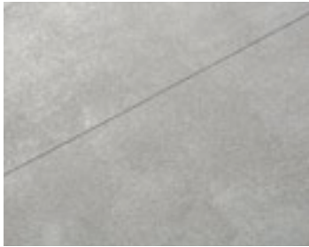
P1: cast-in-place concrete paving with silicon carbide and saw-cut joints
