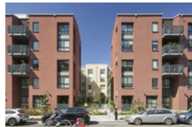
Full-height opening to internal courtyard
