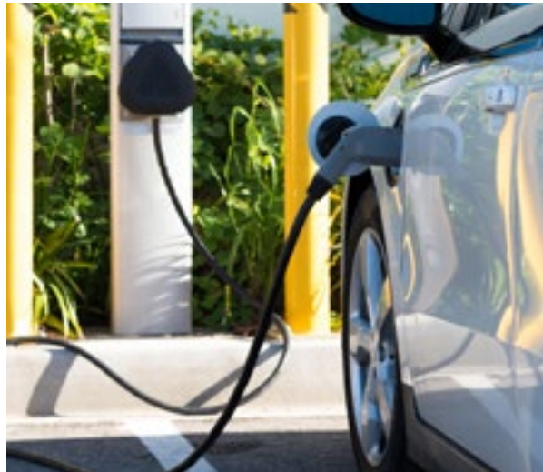
Electric vehicle charging stations
