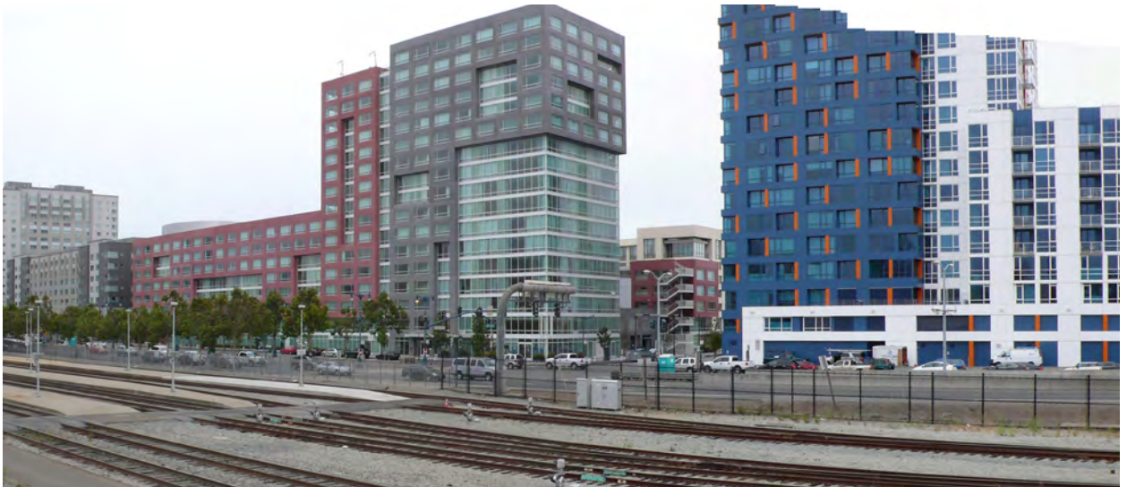
View to the east and south, new residential development along King Street
