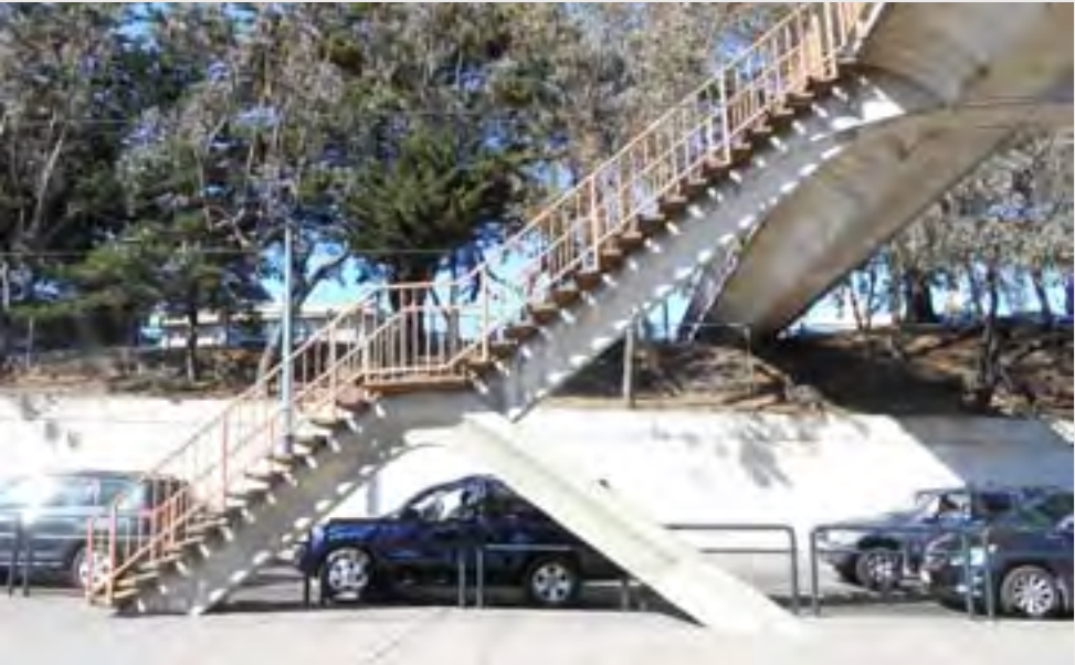
Precast stair treads and steel picket railing at stacked arch columns.
