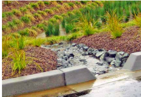
Water diverted from storm drains into a rain garden
