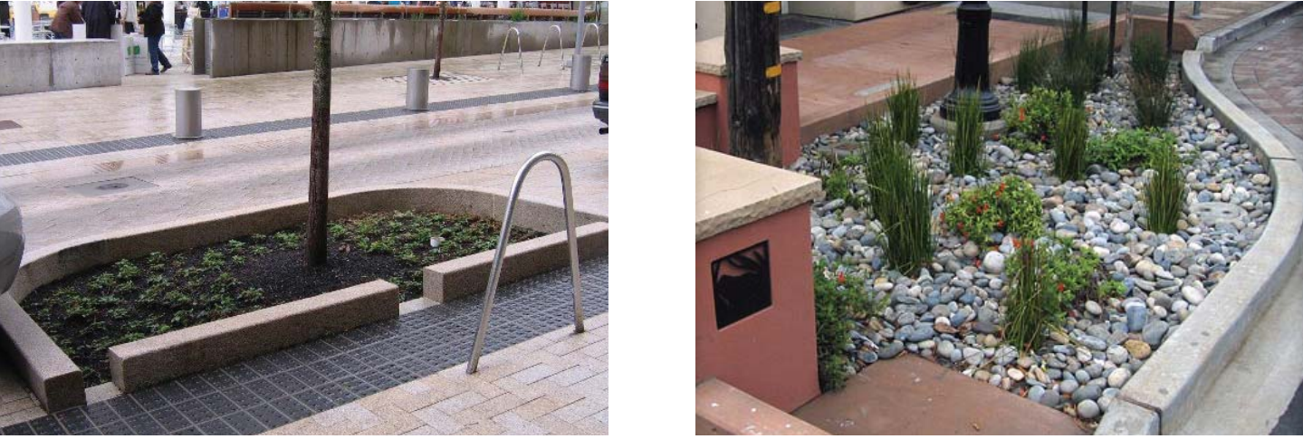
Stormwater infrastructure like bio-retention gardens (rain gardens) can help beautify the streetscape while reducing stormwater runoff.
