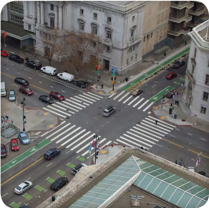
Polk & Grove Intersection
