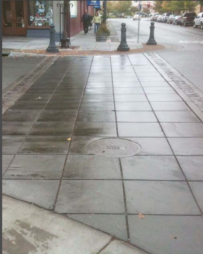
Scored concrete in crosswalk
