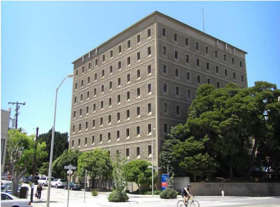
Monteagle Building: View looking northwest from Valencia Street and Duncan Street
