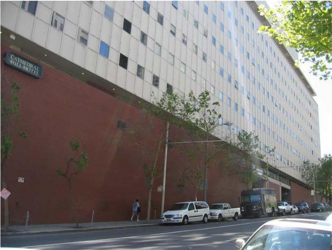
View looking southwest from Post Street
