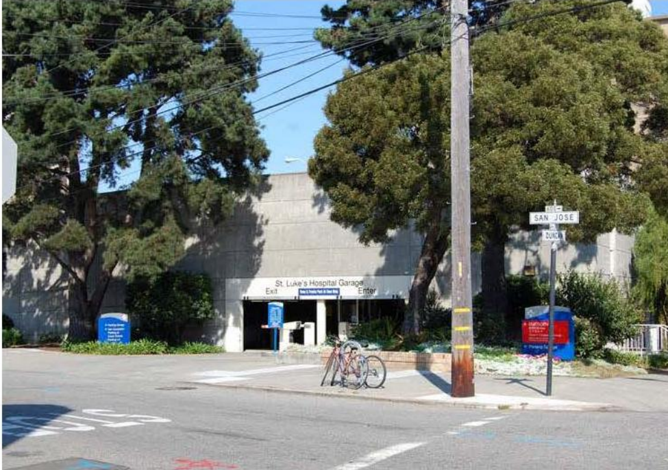
Duncan St. Parking Garage: View looking northeast from Duncan Street and San Jose Avenue
