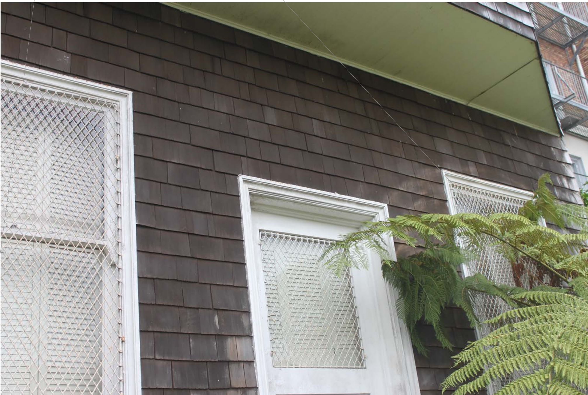
LOWER REAR OF HOUSE
