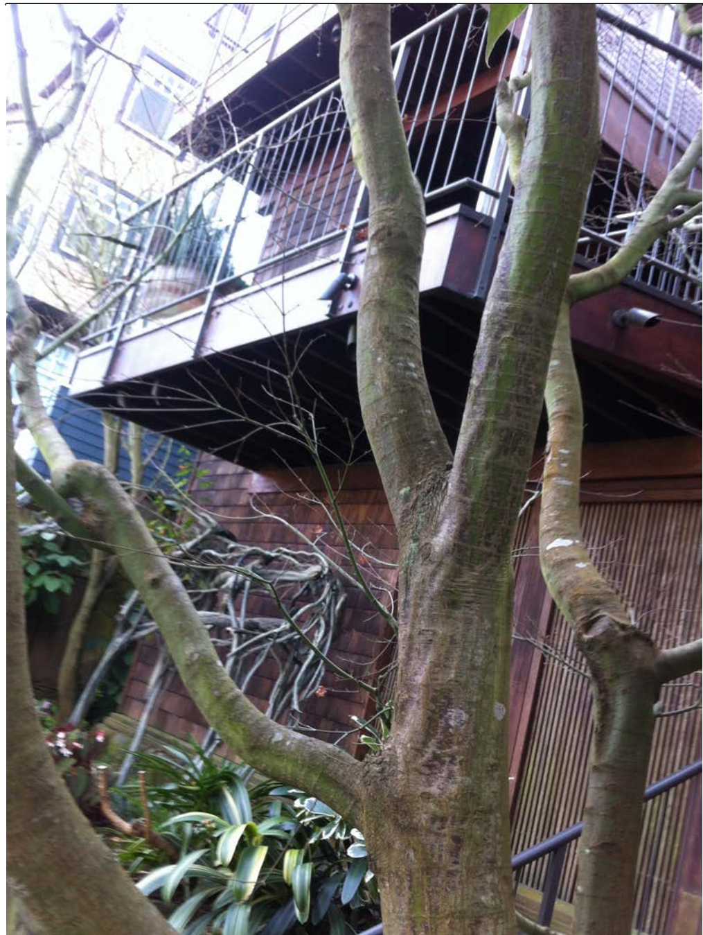
WALL AT LOWER DECK
