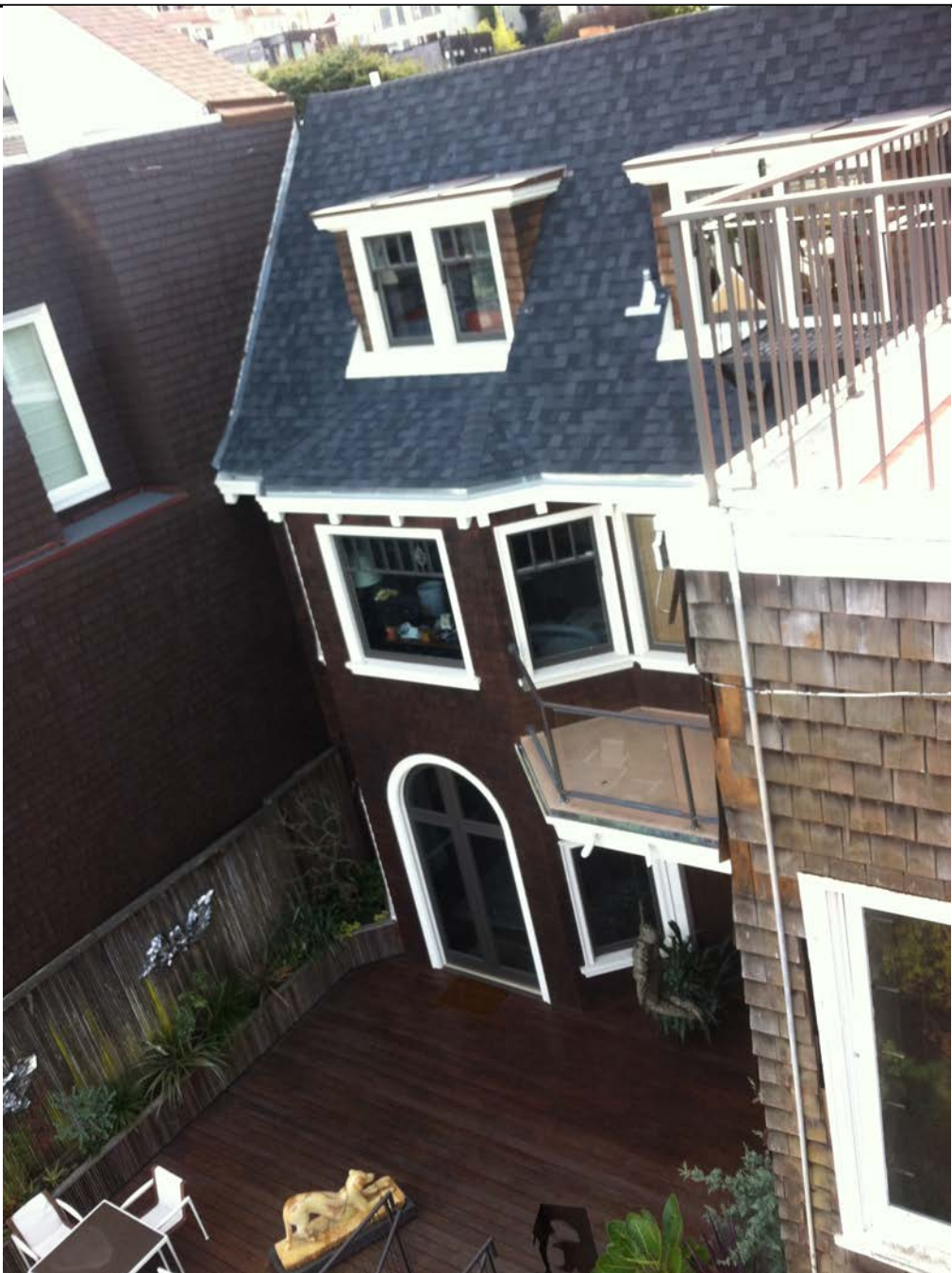
ADJ. PROPERTY REAR FACADE
