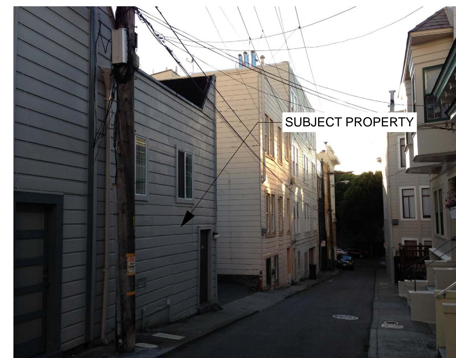
VIEW LOOKING WEST ON LYNCH ALLEY
