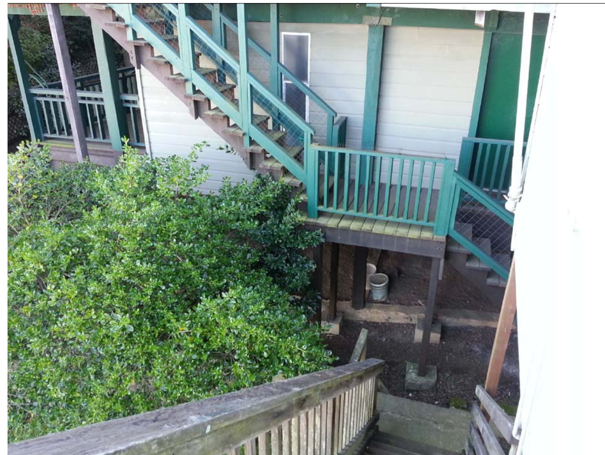
(2) LOOKING SOUTHEAST TOWARD AT 121 MANCHESTER
