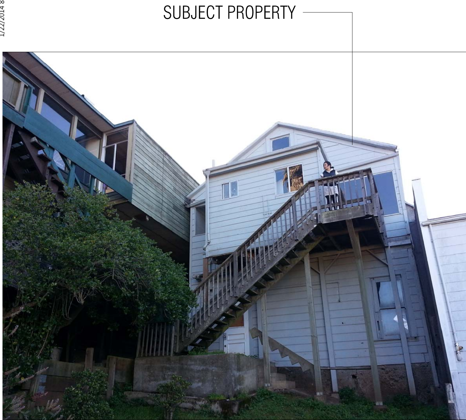
REAR FACADE LOOKING SOUTHWEST
