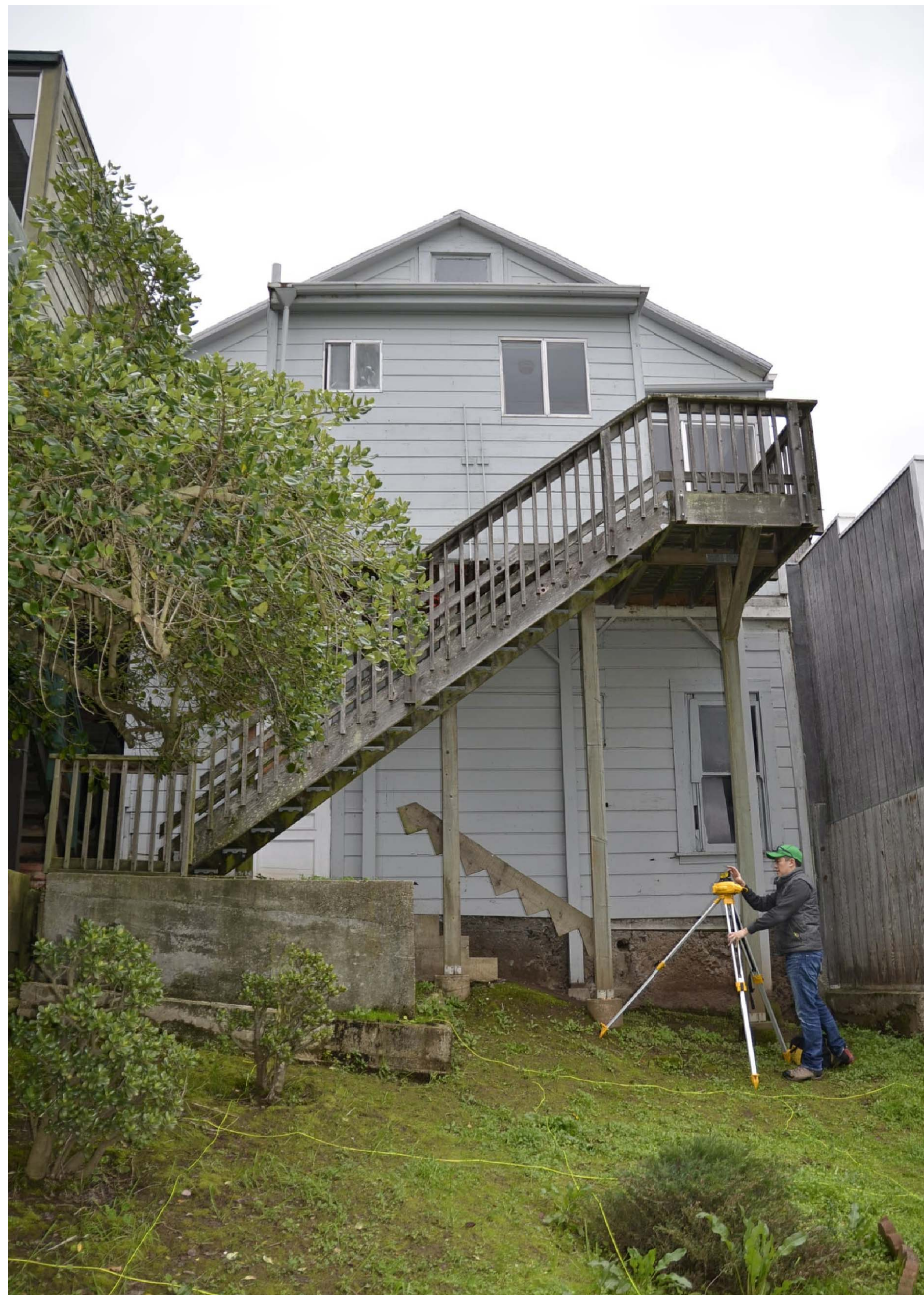
REAR FACADE LOOKING WEST
