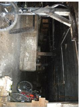
Crawlspace - View East
