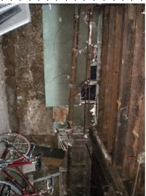
Crawlspace - North Wall
