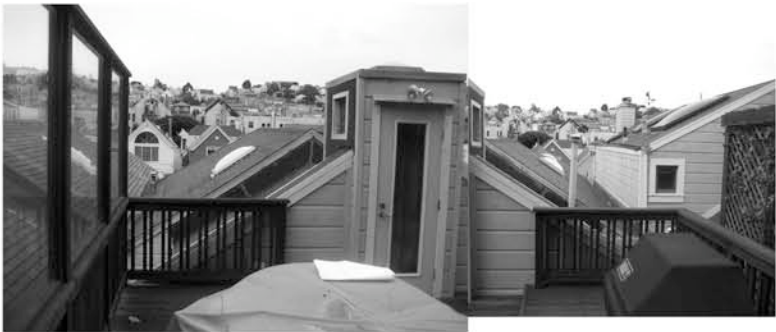
4 REAR DECK OF 309 JERSEY LOOKING NORTH
