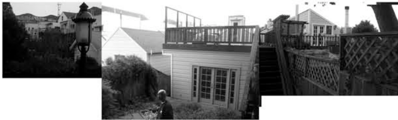
6 BACK YARD OF 309 JERSEY LOOKING NORTH
