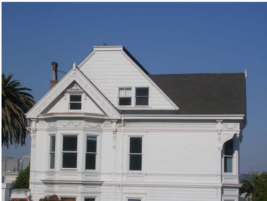
Image 6. West elevation, roof addition for expansion of attic adjacent to original ornamental gable at left. Knapp Architects, digital photograph, 2009.
