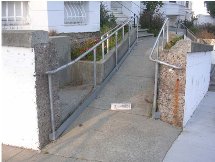
Image 15. Corner of Steiner and Grove Streets, view of original retaining wall that was cut to install a ramp along the south side of building. Knapp Architects, digital photograph, 2009.
