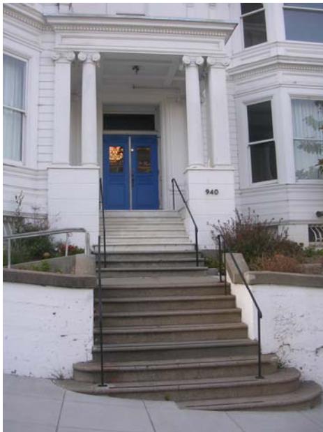
Image 19. At left, the entry porch with Ionic columns. At right, swan-neck pediment decoration above the window openings in each door leaf express the free classic elements within the Queen Anne Style. Knapp Architects, digital photograph, 2009.
