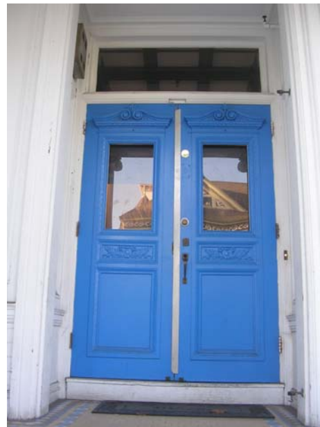
Image 19. At left, the entry porch with Ionic columns. At right, swan-neck pediment decoration above the window openings in each door leaf express the free classic elements within the Queen Anne Style. Knapp Architects, digital photograph, 2009.
