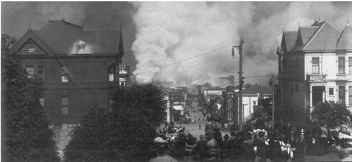
Image 24. At left, 940 Grove Street from Alamo Square during the 1906 Earthquake and Fire of San Francisco. The original upper roof was hipped with a widow's walk. The whitish mass seen at the roof appears to be a chimney on the west side of the main gable roof. The chimney was likely damaged during the earthquake and fell to the ground stripping a gutter below along the way.
