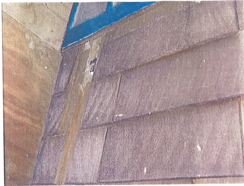
Image 11. Detail of wood shingles, visible at passageway at west side of house. Photo Frederic Knapp, 2007.
