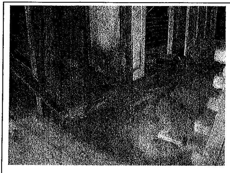
Photo 9: 1 st floor's floor framing set directly into ground. Top of retaining wall is visible in the foreground of the far left photo. Views are facing northeast.
