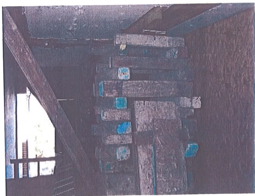
Image 8. Temporary support under the house, looking north to Lombard Street. Photo Frederic Knapp, 2007.
