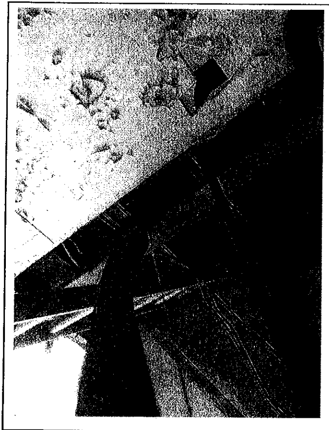
Photo 8: View of the diagonal 2x shoring members from previous photo. View facing upwards along 2x. Notice the straight string line versus the failed and bowed diagonal shoring. The weight of the building has caused the diagonal shoring to warp; shoring has failed.
