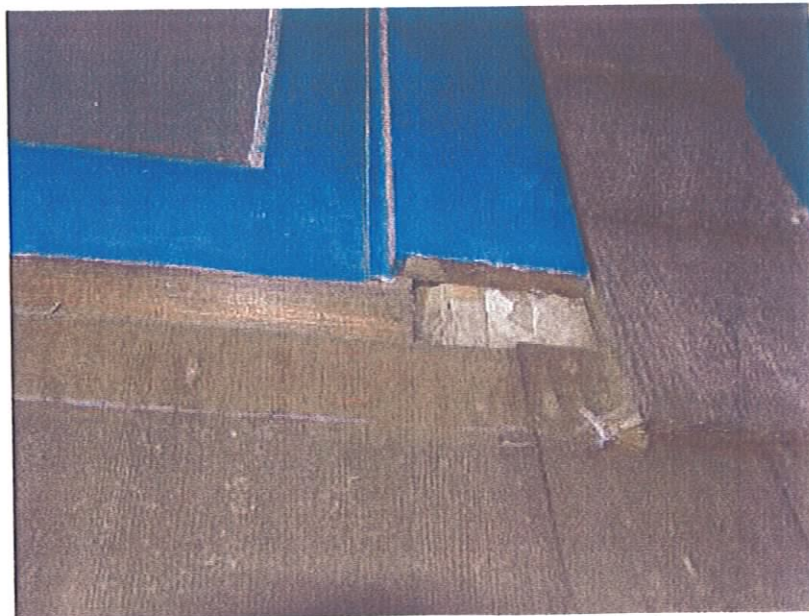
Image 12. Detail of wood shingles at passageway. Note that window trim and shingles are flush. Photo Frederic Knapp, 2007.
