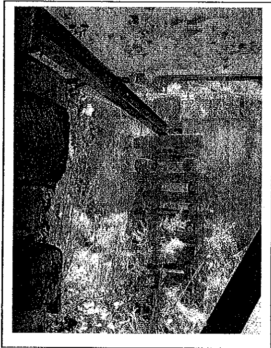
Photo 5: View is from the 1 st floor, taken from the interior of the building facing south. Exterior walls of the 1 st floor are missing, as per previous photo. Notice the minimal 4x4 cribbing members used for shoring, and the rusted steel beam. The backyard's retaining wall is visible in the background.
