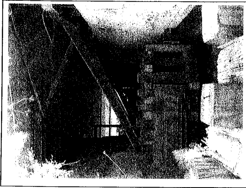
Photo 7: 1 st floor, view is facing north. Notice 1x shoring support post on the far left is braced against the neighbor's exterior stud wall (illegal to lean on neighbor's property). There are minimal 2x diagonal shoring members, bracing back to the shoring cribs.
