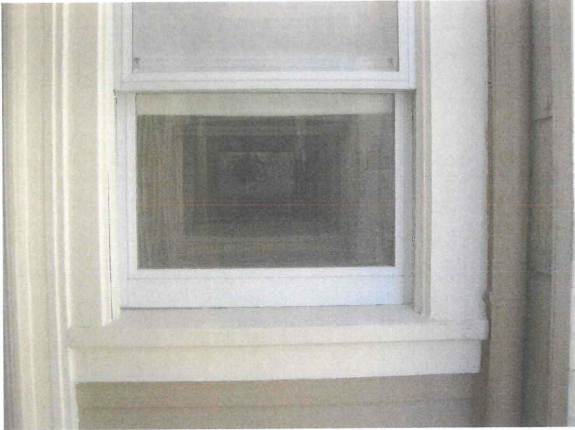
N View, 33 Sutro Hts looking N across light well to bathroom
