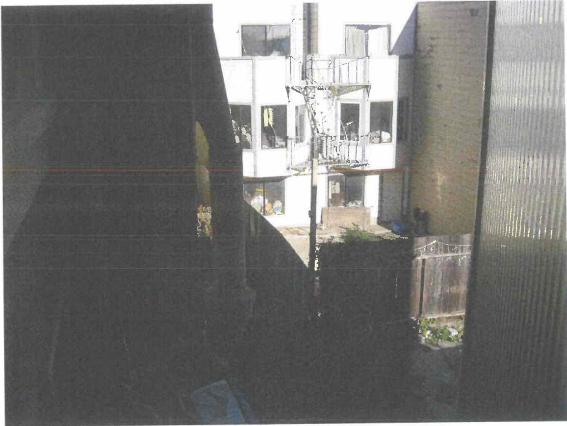
E view 33 Sutro Hts lightwell looking across 27-29 Sutro Hts to 661 46th Av
