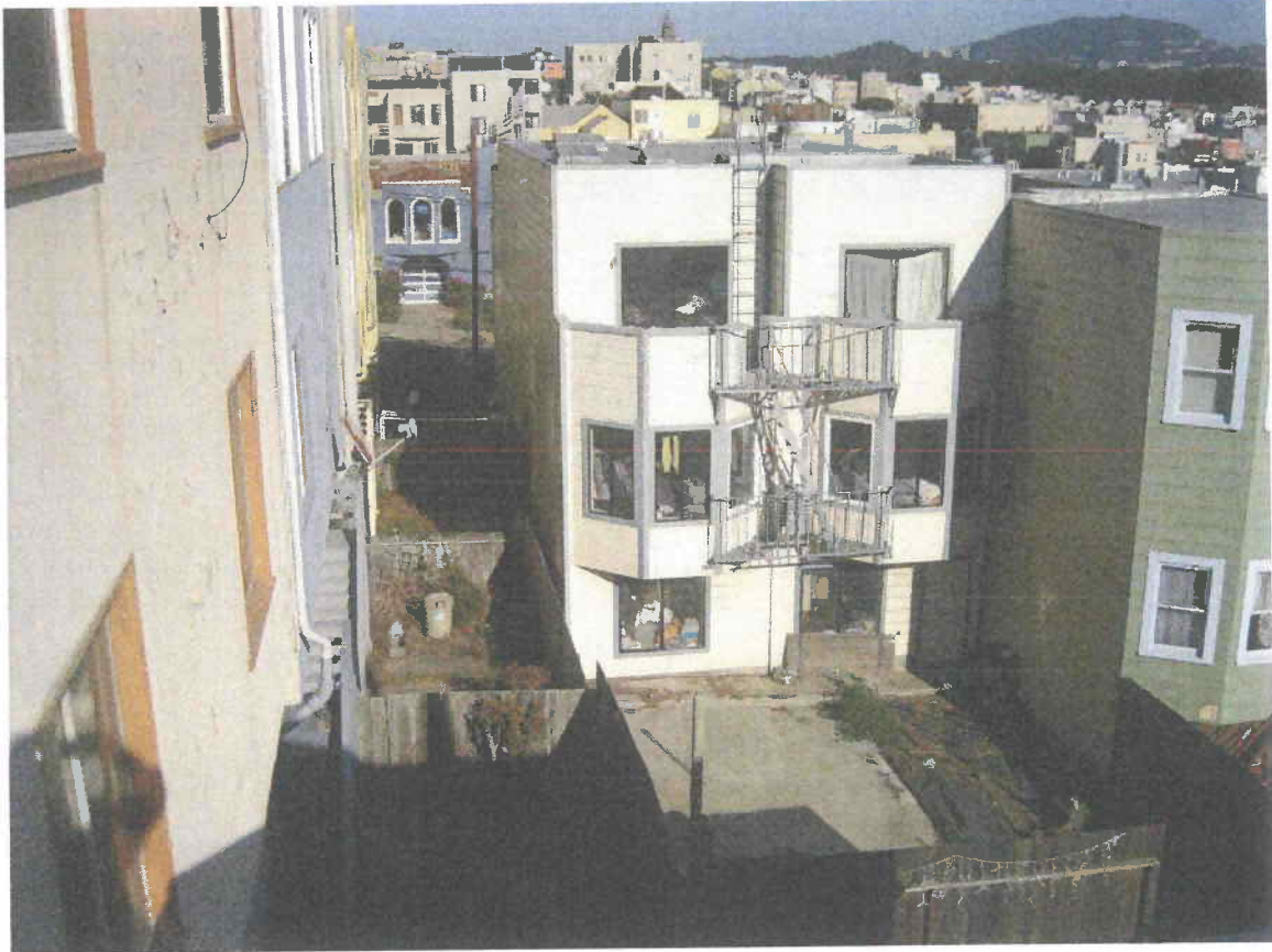
E view from 33 Sutro at roof above light well across 27-29 Sutro Hts along building line to E of 46th Av
