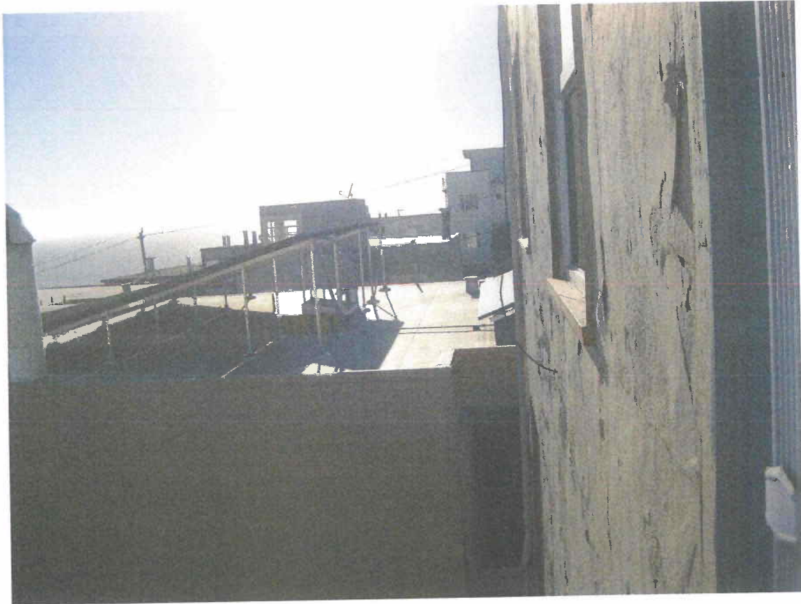
W view from bedroom 23 Sutro Hts across 27-29 Sutro Hts to roof of 33 Sutro Hts and solar arrays
