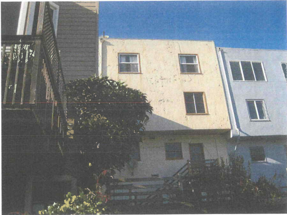
N view from 33 Sutro Hts backyard looking at fence line (left) with privacy tree separating deck and 27-29 Sutro Hts (center), 21-23 Sutro Hts (right)
