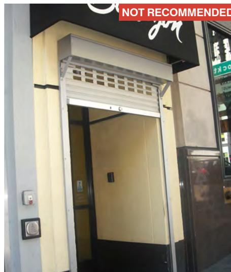
LEFT: When an external security grate is installed, its operational mechanism should be hidden from view. When fully retracted, the security grate should be concealed within the facade or behind the cladding.
