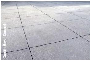
Enhanced Cast-in-Place Concrete with Saw-Cut Joints
