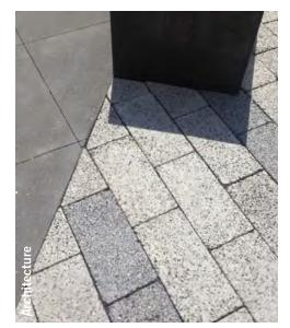
PERMEABLE CONCRETE UNIT PAVERS
