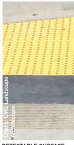
DETECTABLE SURFACE PAVING - SFDPW STAN-DARD
