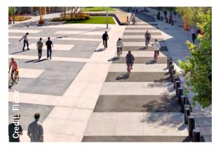
Enhanced Concrete and/or Pre-Cast Unit Pavers with Contrasting Pattern
