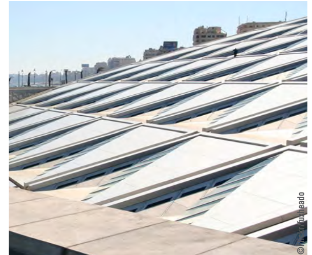
Roof Systems that Enhance Internal Daylighting Alexandria Library / Alexandria, Egypt
