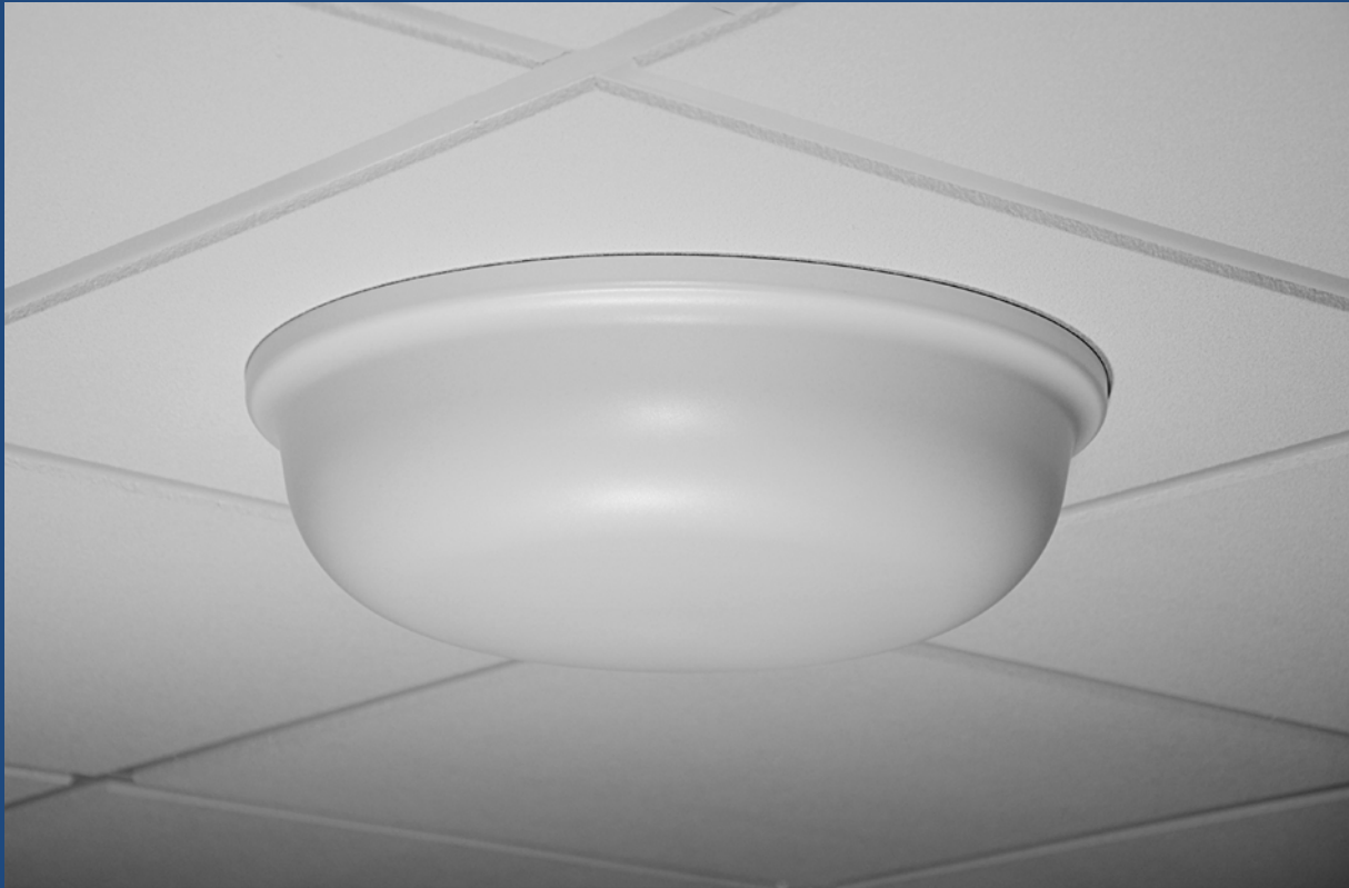
Small (palm-sized) antenna attached to office ceiling
