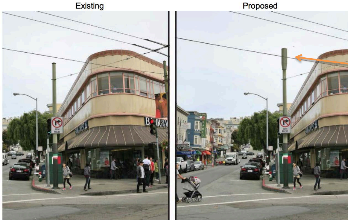
Existing transit pole on the left and a proposed Small Cell (on Columbus Avenue) on the right. The Italian flag tri-colors painted on the existing pole (below sign) would be retained.
