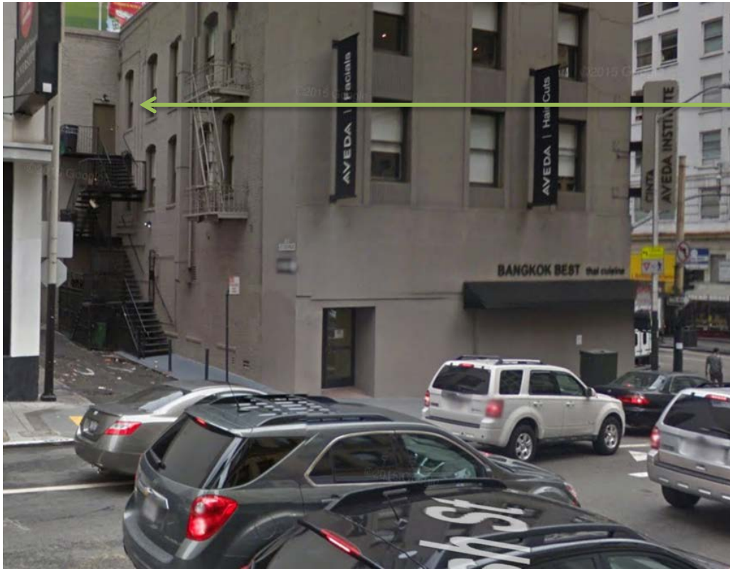
Example of a caged access ladder prominently visible from a surrounding street (disfavored).
