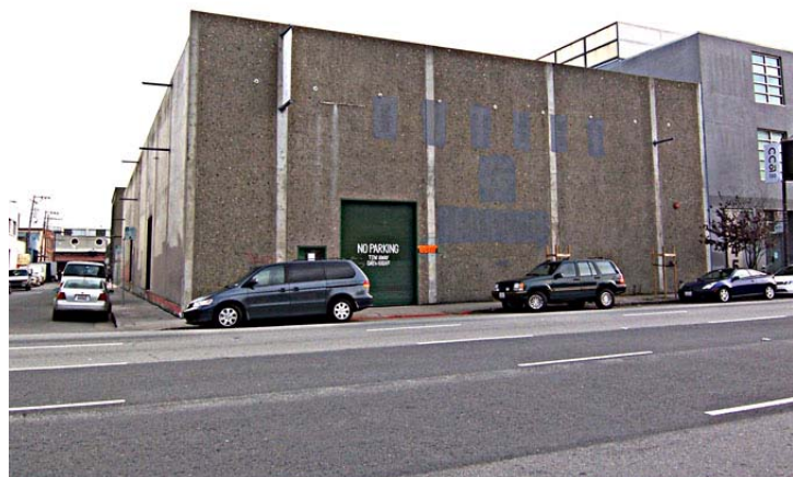
Figure 51. 925 Bryant St. Source: KVP Consulting
