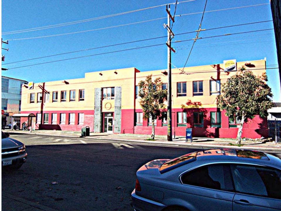
Figure 69. John A. Roebling & Sons Wire Rope Factory, 1740 17 th St. Source: KVP Consulting
