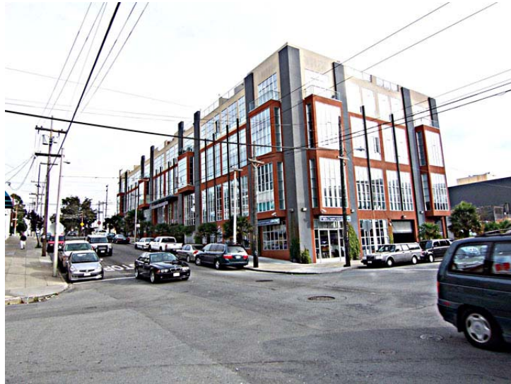
Figure 54. 1800 Bryant St. Source: KVP Consulting
