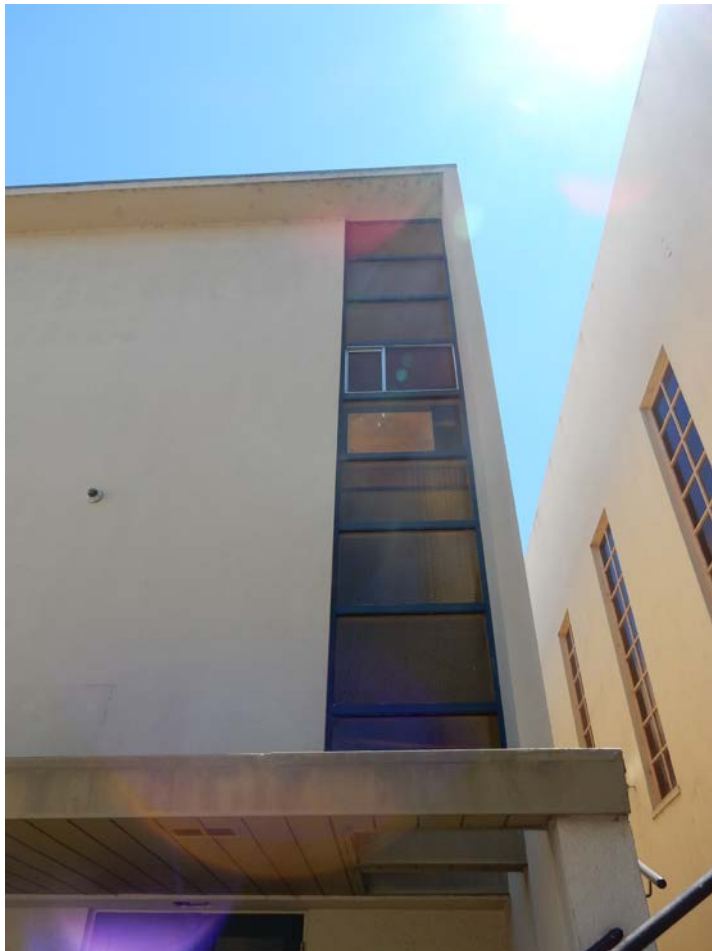
Vertical wood ribbon windows with textured yellow glass on north elevation of youth center and fellowship building, view south.
