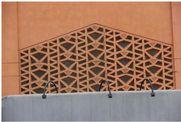
Figure 8. Concrete grille above main entrance.
