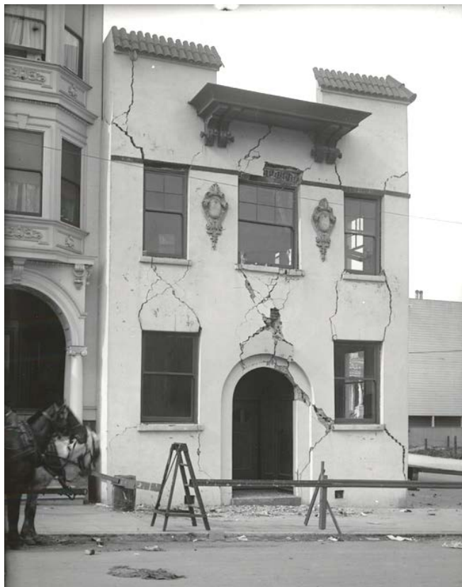
1950-1952 15 th Street, designed by August Nordin and constructed in 1901 as a can factory for Edwin Bennett. This brick masonry building was heavily damaged during the 1906 Earthquake and subsequently replaced. (Bancroft Library)
