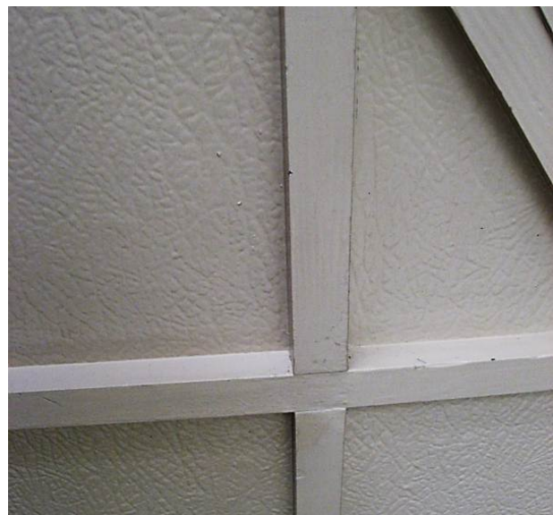
Detail of the leather paper wall cladding
