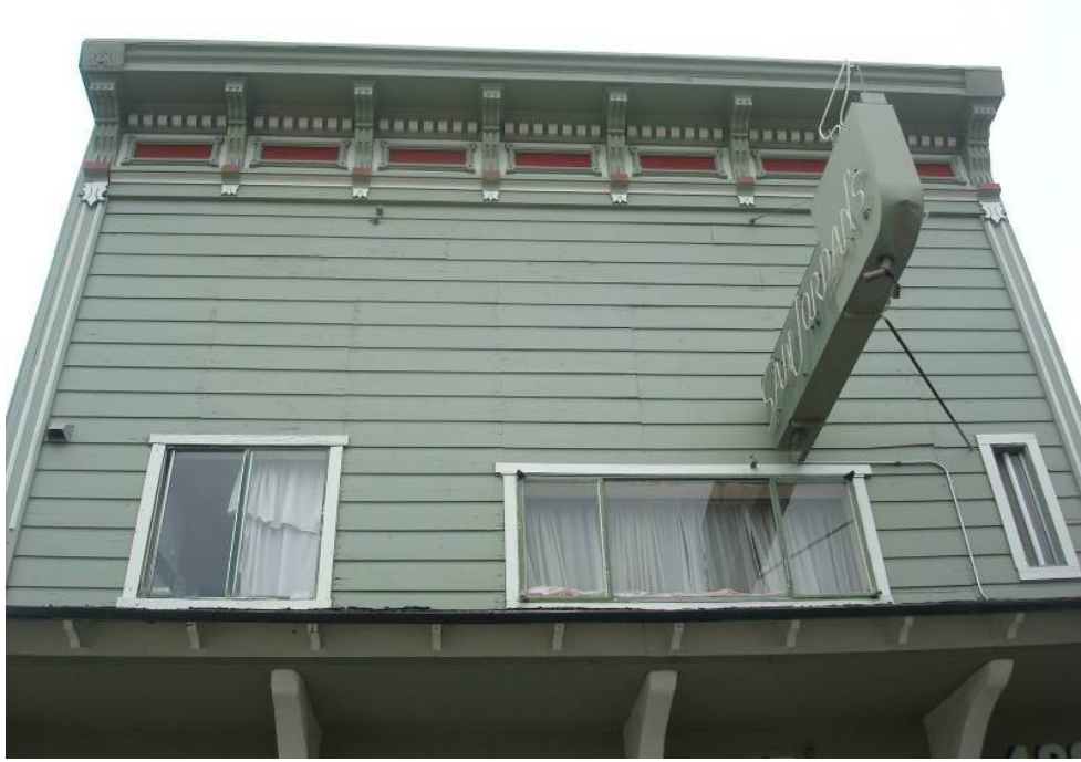
Second story, primary facade.
