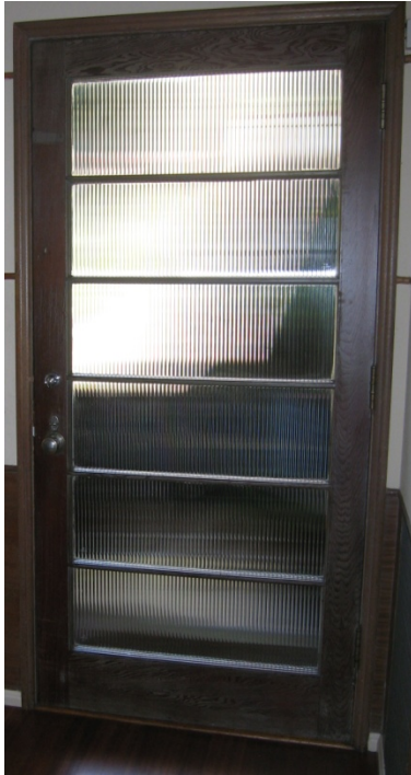
Left: Interior door with ribbed decorative glass set in horizontally oriented muntins (2012).
