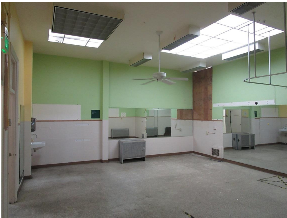
South ward room, view southeast.
