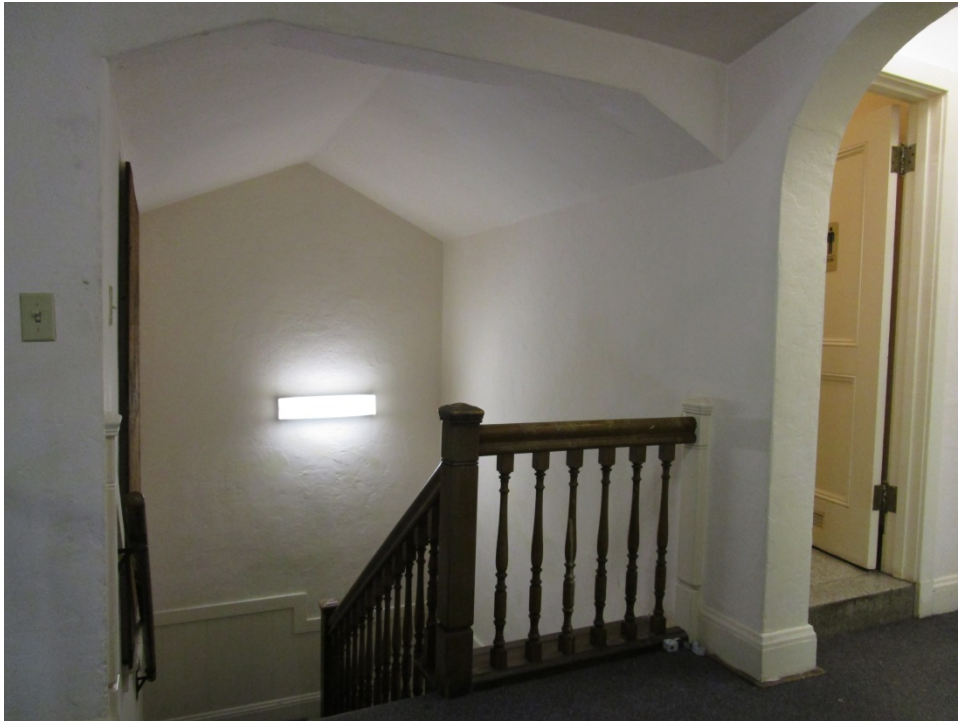
View of stair landing at second floor; note turned wood balusters, vertical board wainscot at staircase, and vaulted ceiling.
