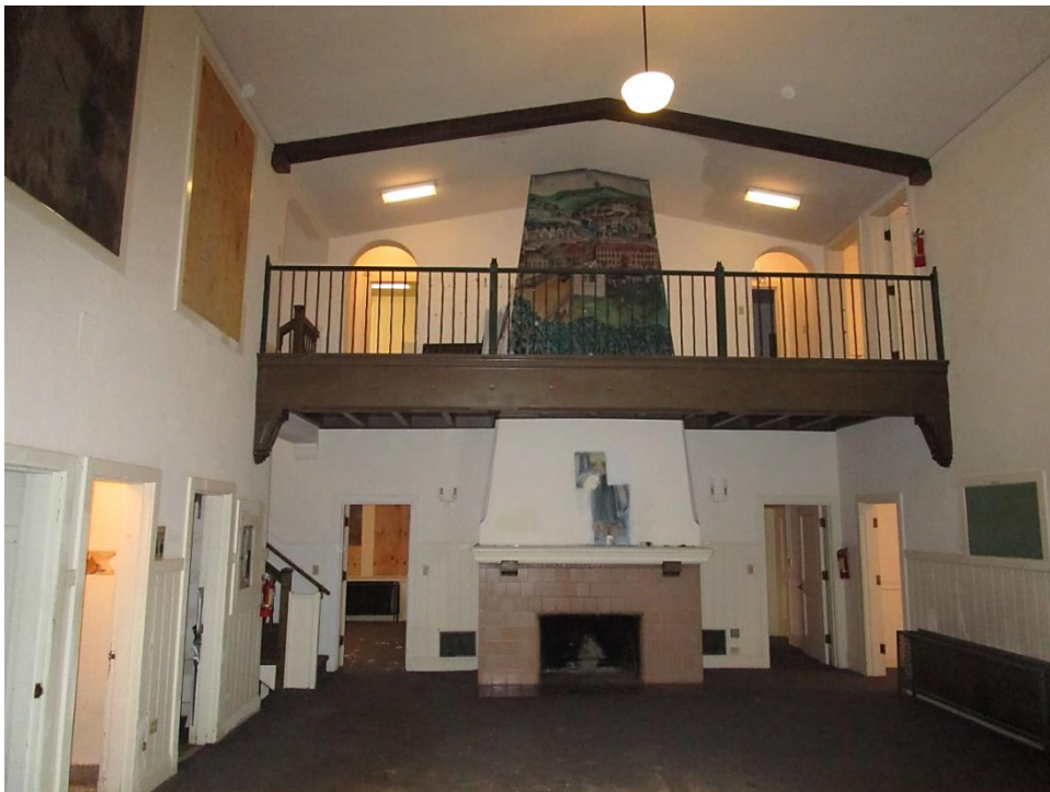
Lobby, view south; note double height volume, gable ceiling with wood beams, balcony, central fireplace with tapered chimney, metal candle scones and openings flanking fireplace and chimney, and vertical board wainscot with flat board trim throughout
