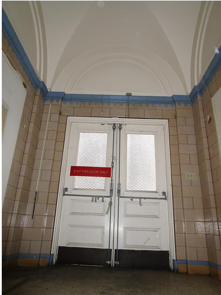
Entry vestibule; note tan-colored wall tiles with blue-colored tile borders, blind arches and a vaulted ceiling.
