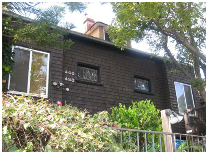
Front façade of the Robins house located at 438-440 Capp Street. View northwest. San Francisco Planning Department.
