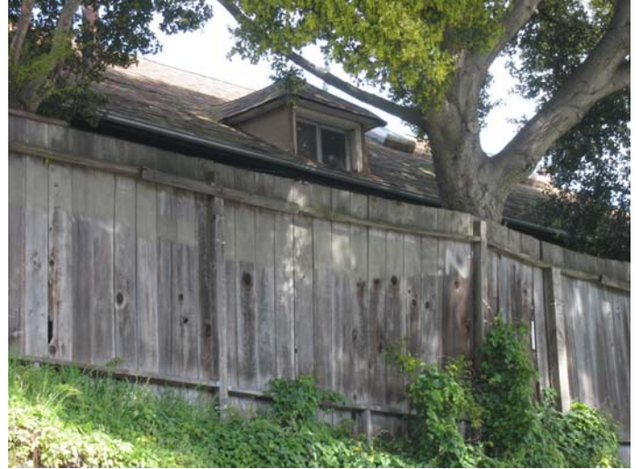
Roof detail at the south side of the Robins house located at 438-440 Capp Street. View northeast. San Francisco Planning Department.
