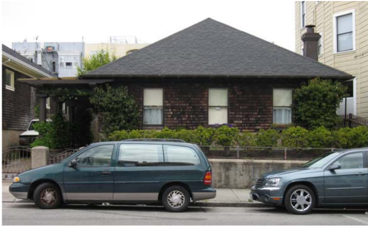
The Wilhelm house located at 426-428 Capp Street. View west. San Francisco Planning Department.
