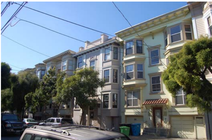
A row of “Romeo” flats located on the west side of Albion Street. View southwest. San Francisco Planning Department.
