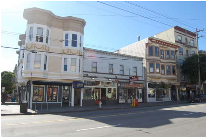
Mixed-use buildings and storefronts located on the south side of 16 th Street. View southwest. San Francisco Planning Department.
