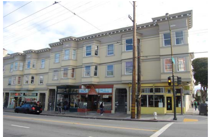
A wide commercial frontage that is divided into multiple small storefronts located on the south side of 16 th Street. View southeast. San Francisco Planning Department.
