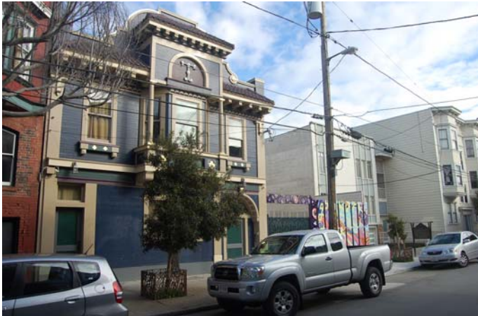
The social hall located at 141-143 Albion Street. View southeast. San Francisco Planning Department.
