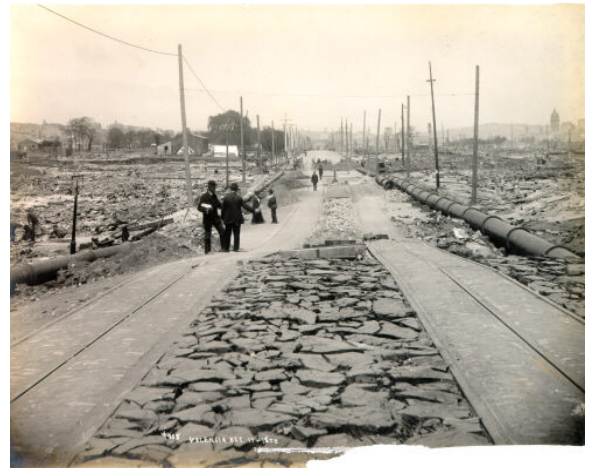
Valencia Street in the aftermath of the 1906 earthquake and fires. View north from approximately the same location as in the photograph to the left. There was total destruction of structures, roads, transit lines, and utility lines. San Francisco History Center, San Francisco Public Library (Historical Photograph Collection Photo Id# AAC-3252).
