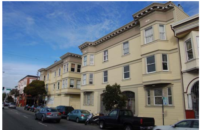
The Henry Gutzeit complex located on the east side of Guerrero Street. View northeast. San Francisco Planning Department. Required information
