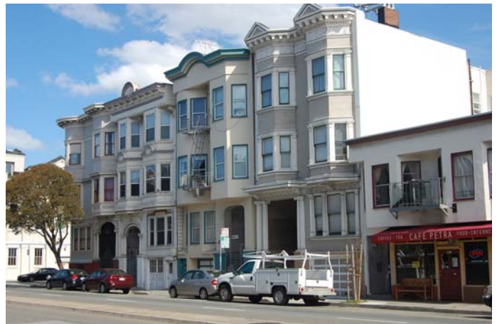
Examples of residential buildings located on the east side of Guerrero Street. View northeast. San Francisco Planning Department.
