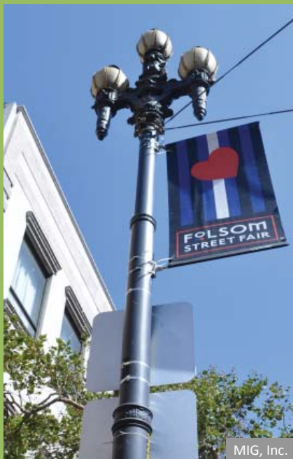
Market St Path of Gold street light with globe luminaires on cast iron post. Dates to 1915.
