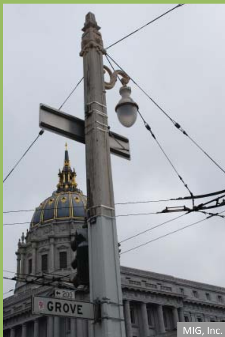
Van Ness single pendant luminaire on a trolley pole at Symphony Hall. Dates to 1915 and 1936.
