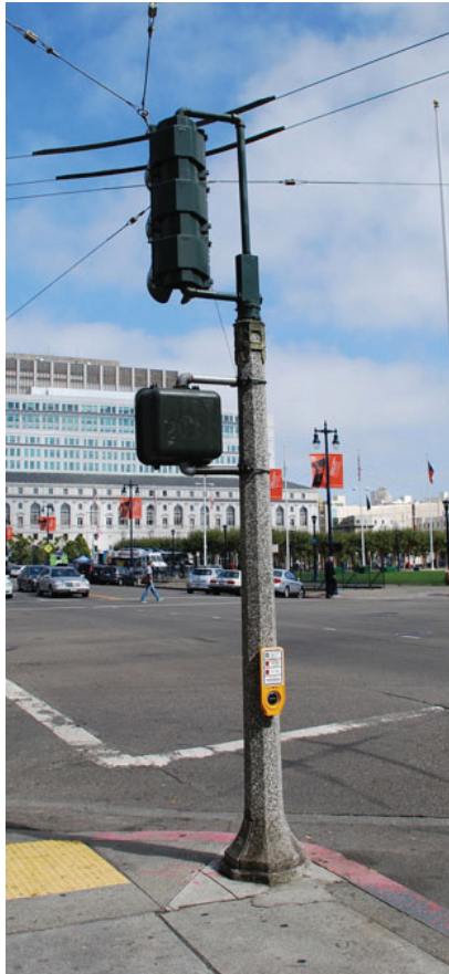
Modified aggregate concrete post with traffic signal
