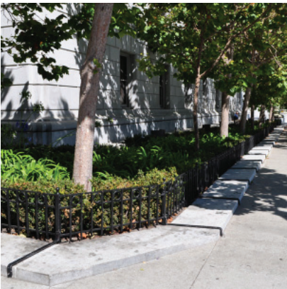
Wide granite planter edging with anchored metal skateboard guards at McAllister St
