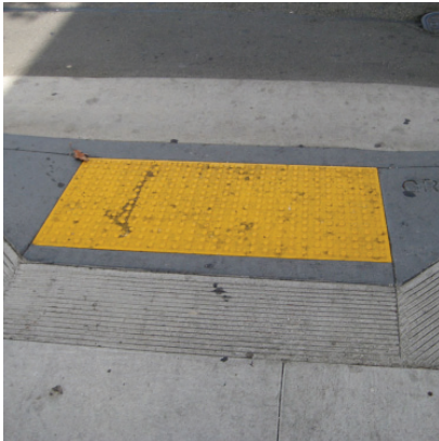
Accessible ramp with truncated domes
