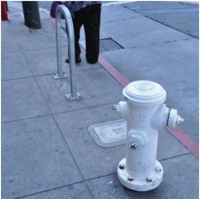
Low pressure hydrant along Larkin St
