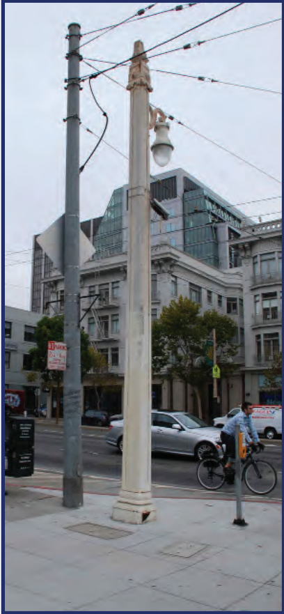
Van Ness trolley pole with single pendant
