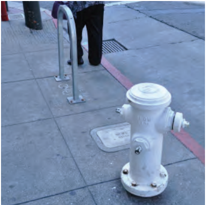
Low pressure hydrant along Larkin St
