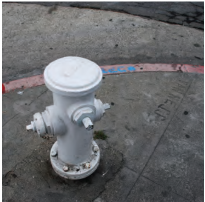
Low pressure hydrant at Redwood St
