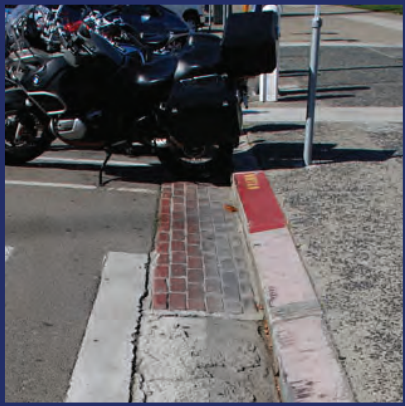
Granite curb with brick gutter along Dr. Carlton B. Goodlett Place
