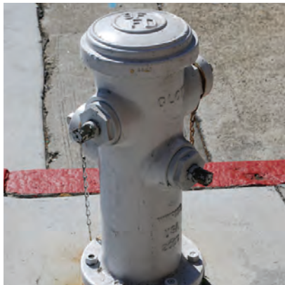
Low pressure hydrant along Franklin St
