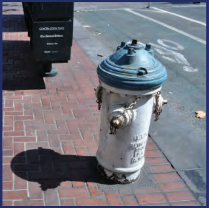
High pressure auxiliary water supply hydrant along Market St
