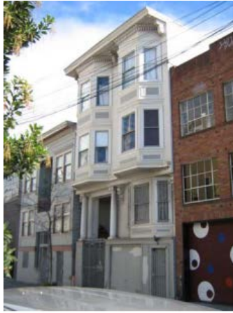
Classical Revival style flats at 439-441 Tehama Street (1906)
