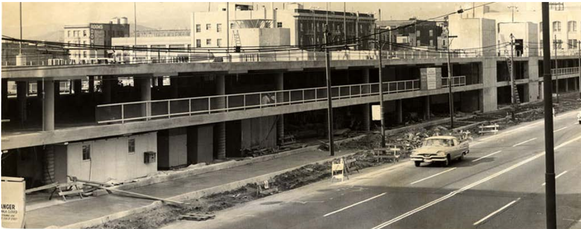
View southwest along Mission Street during construction of the new 5th and Mission parking garage, 1958. (San Francisco Public Library Historical Photograph Collection, AAK-0360)
