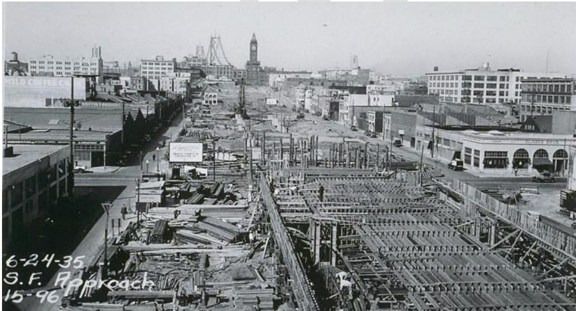
Construction of the Bay Bridge approach, 1935. View is east from near 2nd Street. (U.C. Berkeley Bancroft Library via Calisphere)
