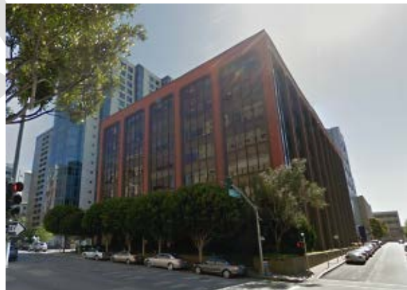
Modern style commercial building at 633 Folsom Street (1966)
