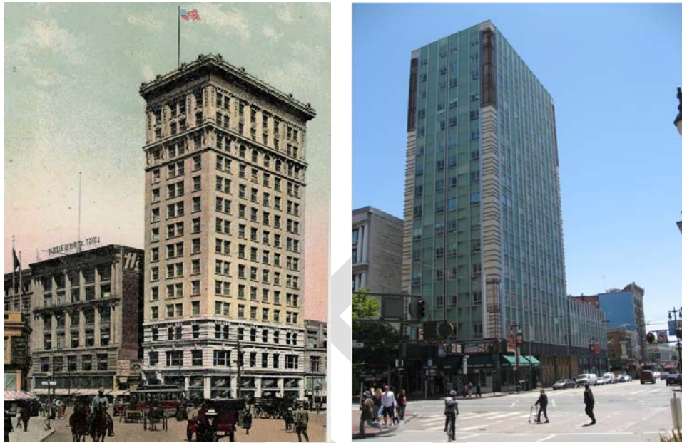
Two views of the David Hewes Building at 6th and Market streets. At left, the building circa 1910. At right, the building in 2013. (Postcard, private collection; San Francisco Planning Department)
