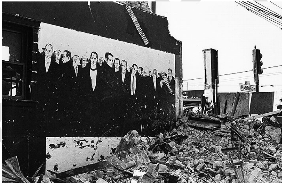
Demolition of the Tool Box showing a mural of leathermen painted by Chuck Arnett, 1971. (FoundSF.org, “Folsom Street: The Miracle Mile)
