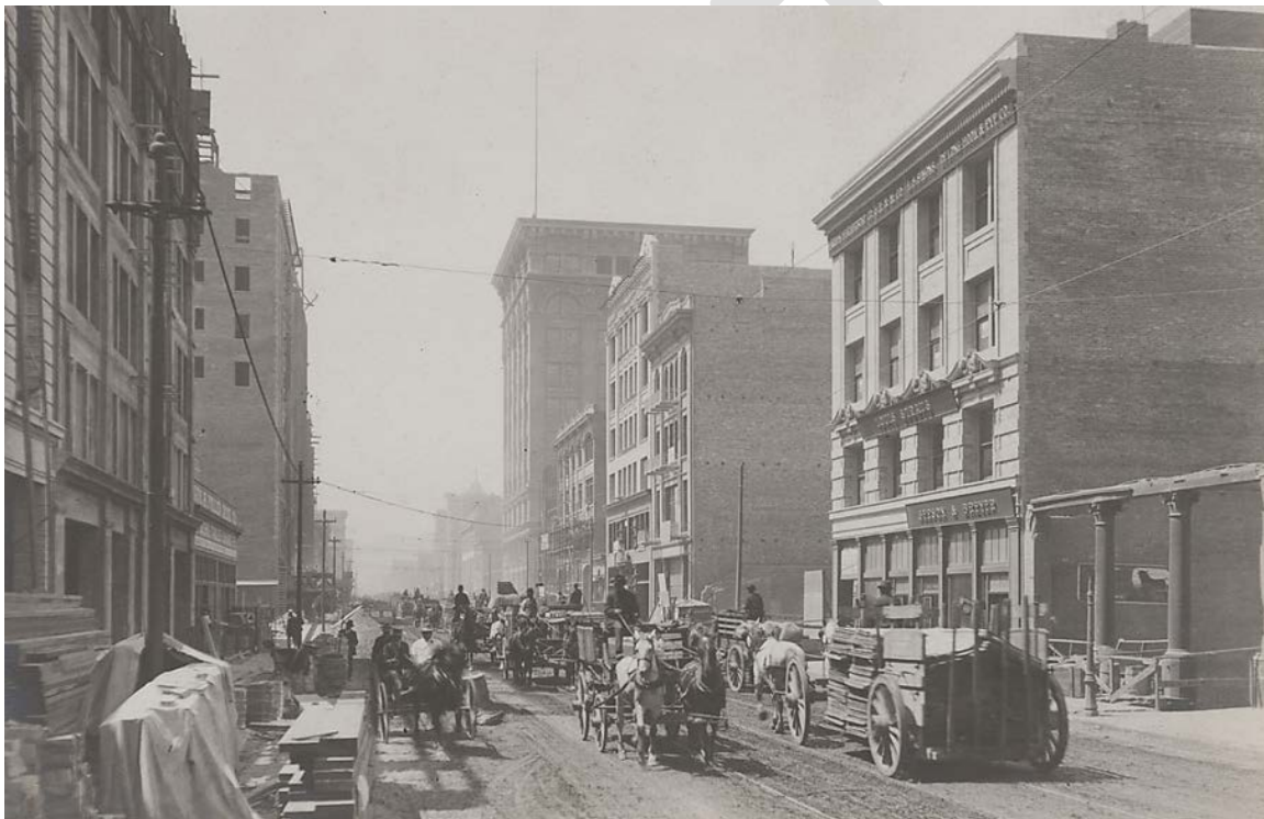
View west along Mission Street between 2nd and 3rd streets, 1907. Note the rapid pace of reconstruction. (California Historical Society)
