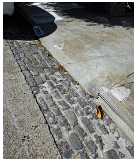
Figure 169 – Basalt block paving in gutter visible between concrete curb and concrete street, near 300-306 Caselli Avenue. (Photo by M.R. Corbett, 5 October 2015)
