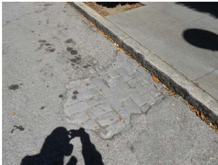
Figure 87 – Deteriorating asphalt paving revealing basalt paving blocks, also granite curb and concrete sidewalk in front of 7 Corbett Avenue. (Photo by M.R. Corbett, 2 July 2012)
