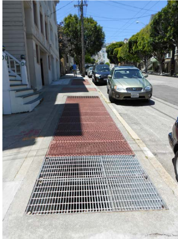
Figure 110 – Ventilator grates over Twin Peaks Tunnel in 4500 block of Eighteenth Street. (Photo by M.R. Corbett, 6 June 2012)
