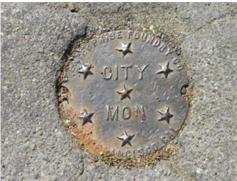
Figure 166 – Hand hole cover for a City Monument, end of Saturn Street, manufactured by Enterprise Foundry Company, date unknown. (Photo by M.R. Corbett, 23 July 2012)
