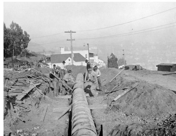
Figure 122 – Building 24-inch sewer pipe on Corbett Road looking north toward Corbett Heights, ca. 1921. (San Francisco History Center, San Francisco Public Library. AAB-3461)
