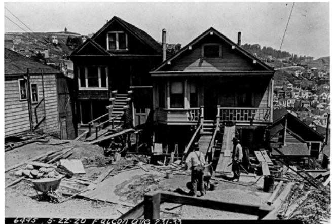
Figure 136 – Houses on Falcon Avenue being moved for Market Street extension, 1920. (Courtesy of Western Neighborhoods Project. Labeling consistent with Department of Public Works Photos.)
