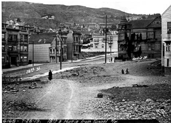
Figure 111 – View west toward Eighteenth and Hattie Streets in 1919 showing clearance of the right-of-way for construction of the Twin Peaks Tunnel and the Market Street extension. (Courtesy of Western Neighborhoods Project. Labeling consistent with Department of Public Works Photos.)
