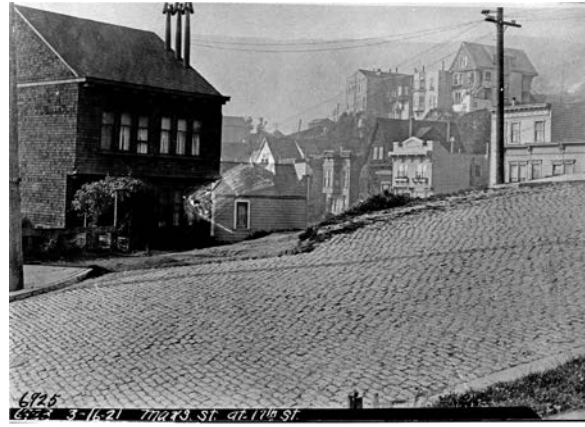
Figure 44 – 1921 view of basalt block paving at Mars and Seventeenth Streets. (Courtesy of Western Neighborhoods Project. Labeling consistent with Department of Public Works Photos.)
