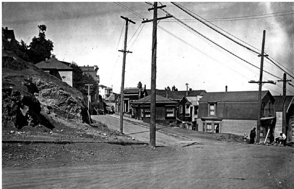
Figure 33 – 1916 view of Roosevelt and Seventeenth Streets showing infrastructure systems: utility poles and wires for telephone and electricity, fire hydrant, stone curbs, workmen with basalt paving blocks. (Courtesy of Western Neighborhoods Project)
