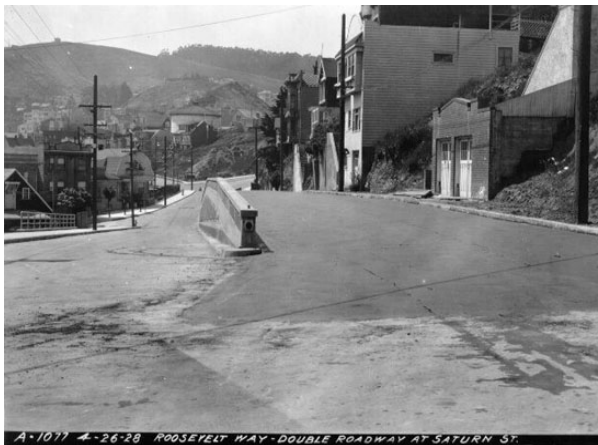
Figure 104 – 1928 view looking south along Roosevelt Way at Saturn showing roadway retaining wall. (San Francisco History Center, San Francisco Public Library. AAB-5162)
