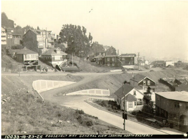
Figure 102 – 1925 view looking northeast at Roosevelt Way showing new concrete retaining walls. (San Francisco History Center, San Francisco Public Library. AAB-5168)
