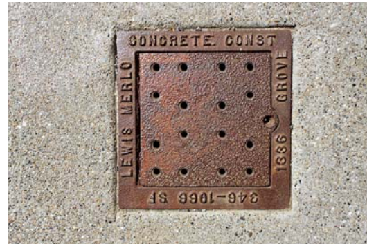
Figure 167 – Hand hole cover for unknown utility near 254 Romain Street. (Photo by M.R. Corbett, 5 October 2015)
